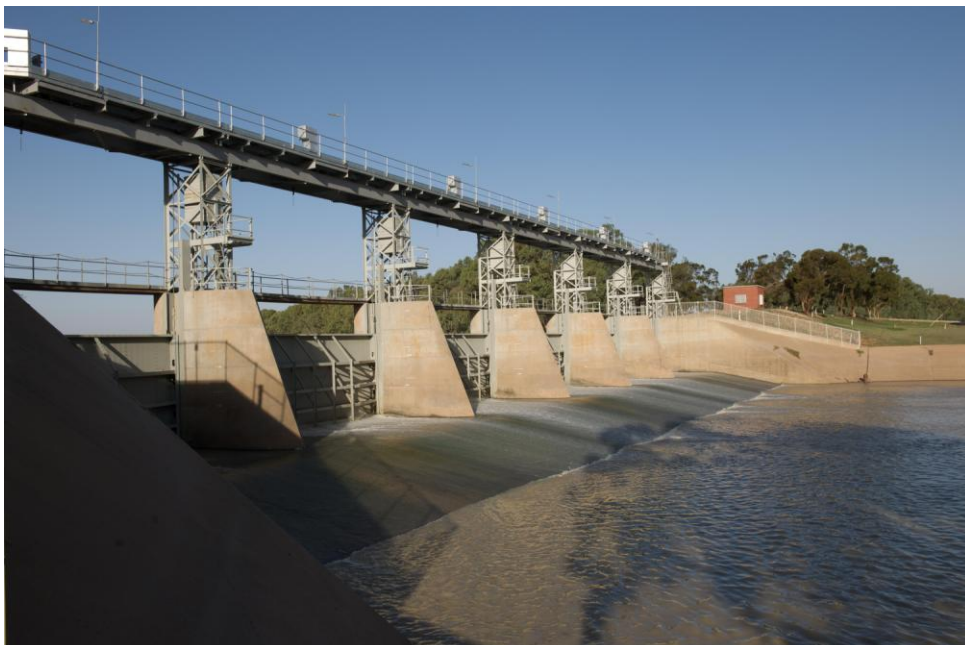
Menindee Weir — water is held back here to fill lakes Pamamaroo and Wetherell. The flood peak reached the Menindee Lakes in early May 2010, increasing their storage level to 88% capacity (photo by Arthur Mostead © MDBA)
