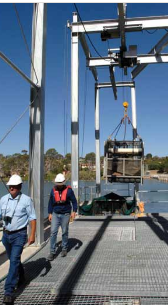
Fishway and carp separation trap on the River Murray at Lock 1, Blanchetown, South Australia. Native fish can swim through, while carp are caught and processed for bait to be used in the fishing industry
