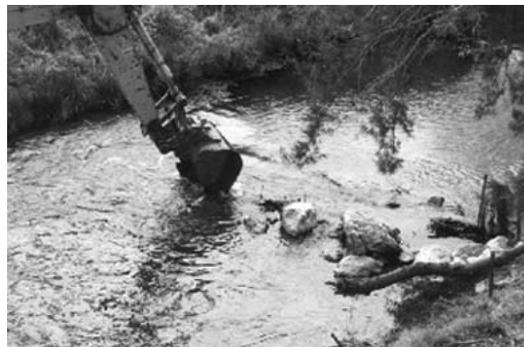
*Figure 3. Removal of unauthorised weir structure, Cudgegong River*
