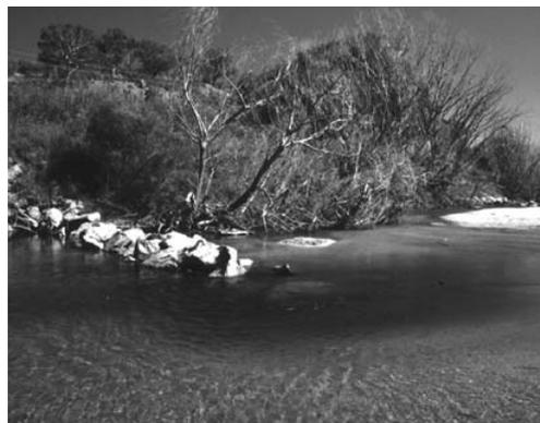
Figure 10. The scour pool at the end of deflector No. 3. Note the sand depositing downstream of the scour pool
