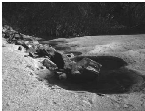
Figure 12. Deflector No. 10 which has been swamped by sand
