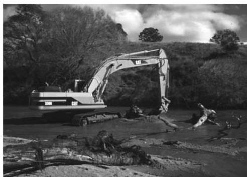
*Figure 7. Excavation of the habitat pool and placement of logs. Note the shallow water the excavator is standing in, indicative of the general depth of the river prior to rehabilitation*
