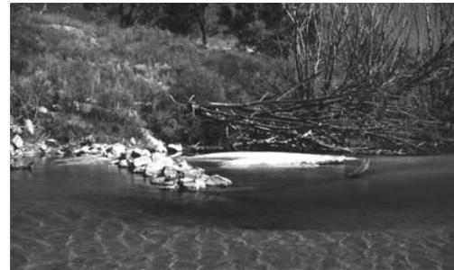
Figure 13. The scour pool of deflector No. 12. Note the snag near the tip of the deflector is still within the pool, whilst the snag in the middle of the deflector has been buried by sand. (see Figure 6 for how the deflector looked immediately after construction)
