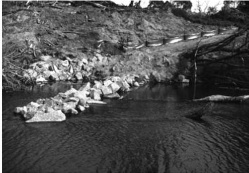
*Figure 5. Completed deflector showing logs projecting downstream. The commencement of rock armouring of the bank can be seen to the left of the deflector*
