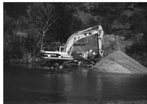
Figure 4. Construction of a deflector from the bank. Note the bank disturbance which has to be stabilised and revegetated.
