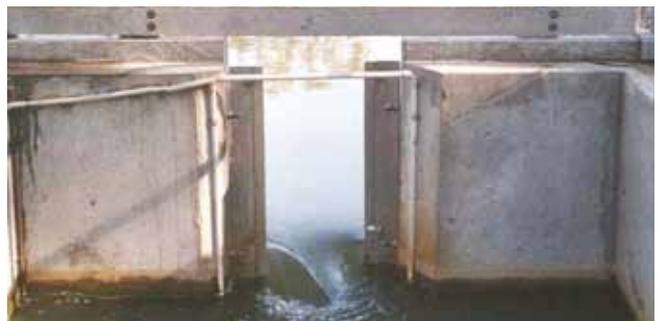
*Upstream exit of the fishway on Lock 8 near Mildura. Both upstream and downstream entry points are fitted with antennas that detect the movements of PIT tagged fish as they pass through the fishway. Image courtesy: Lee Baumgartner NSW DII*
