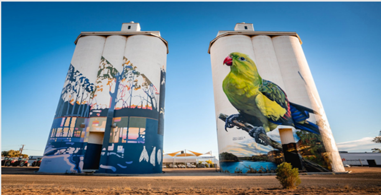
The work of Garry Duncan (on the left) and Jimmy Dvate (right) on the Waikerie silo site on the south bank of the River Murray, in the Riverland region of South Australia. Photo courtesy of Waikerie Silo Art.
