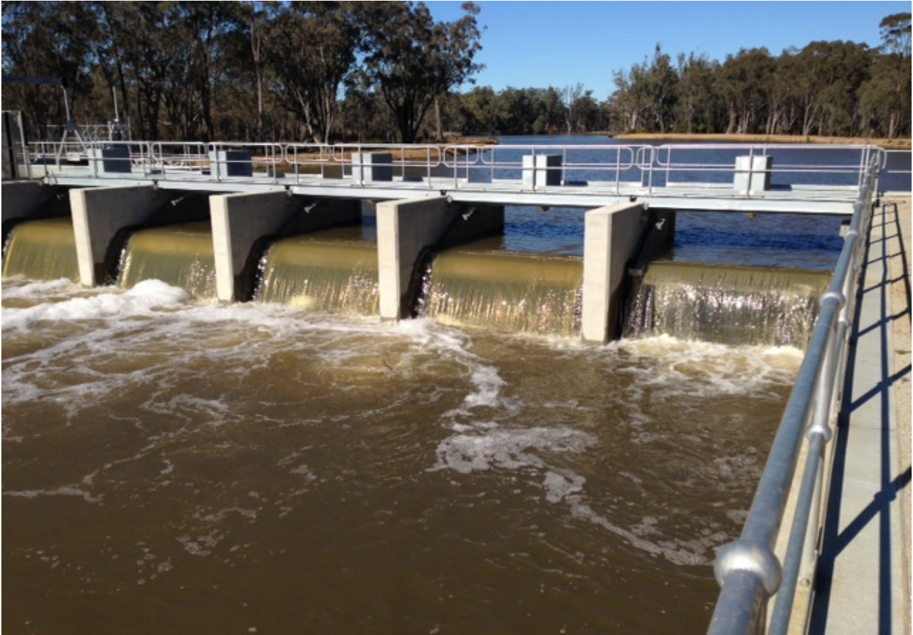
Figure 1 – Water flowing through the new inlet regulator into Koondrook-Perricoota Forest. Around 500 ML/day is passing through the inlet, spread across five gates and two fishways (not visible in photo) (Source: Graeme Hind, State Water Corporation).
