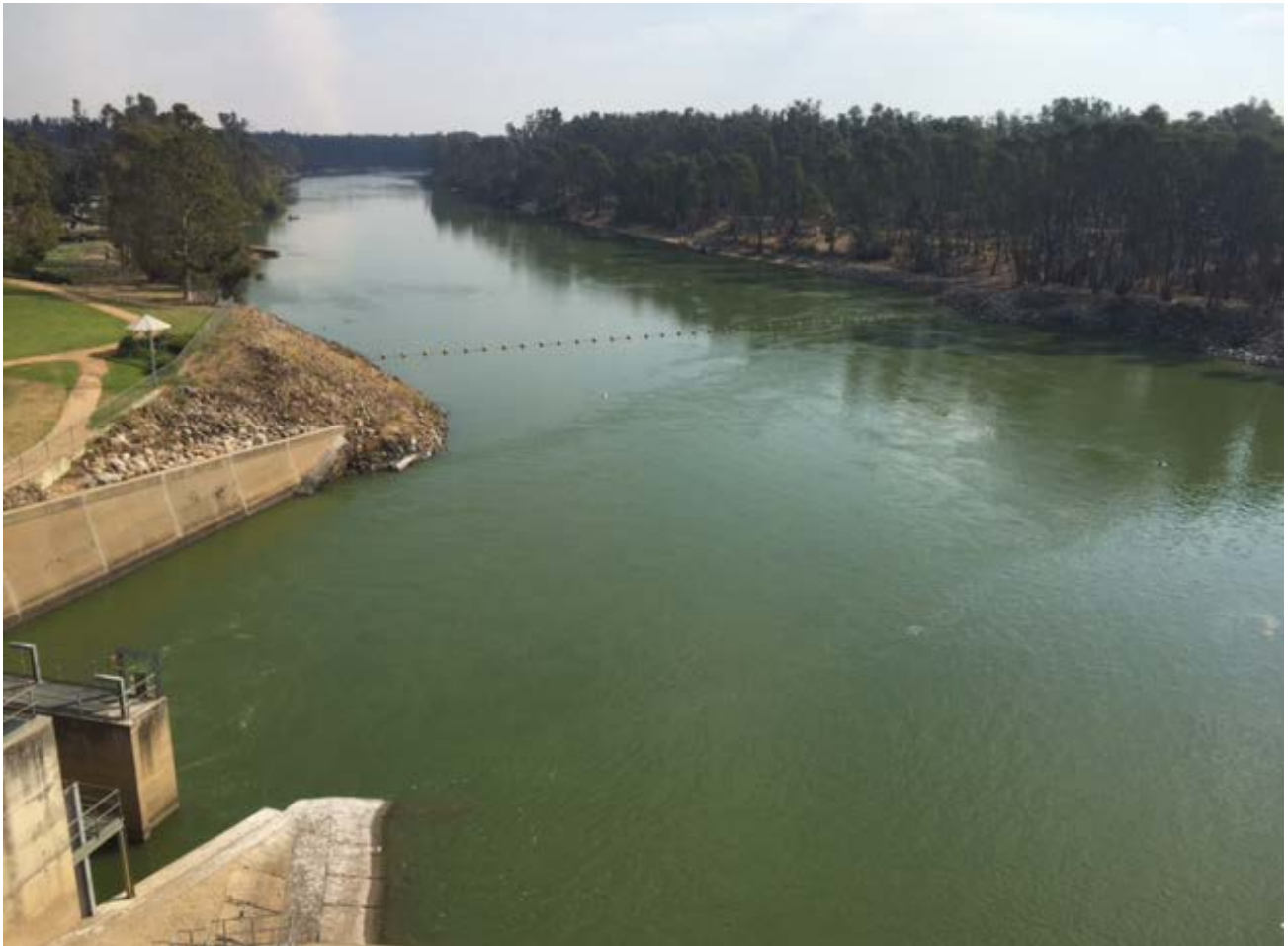
Photo 1 – Looking downstream from Yarrowonga Weir. The current release of 7,000 ML/day is being used to generate hydroelectricity, and can be seen exiting the power station to the left of the above picture. (Source: Luke Cruikshank, Goulburn-Murray Water)
