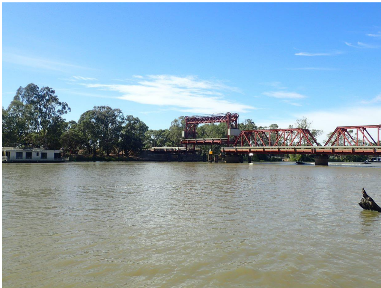
Photo 1 Paringa Bridge in operation on the River Murray at Paringa South Australia. Photos: Tyson Milne
