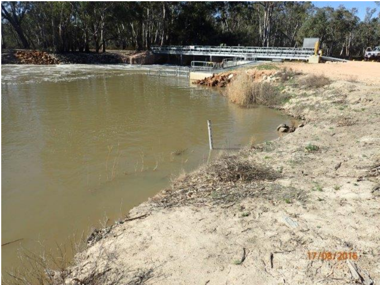
Photo 1 – Flow downstream of pipeclay weir (source SA Water).
