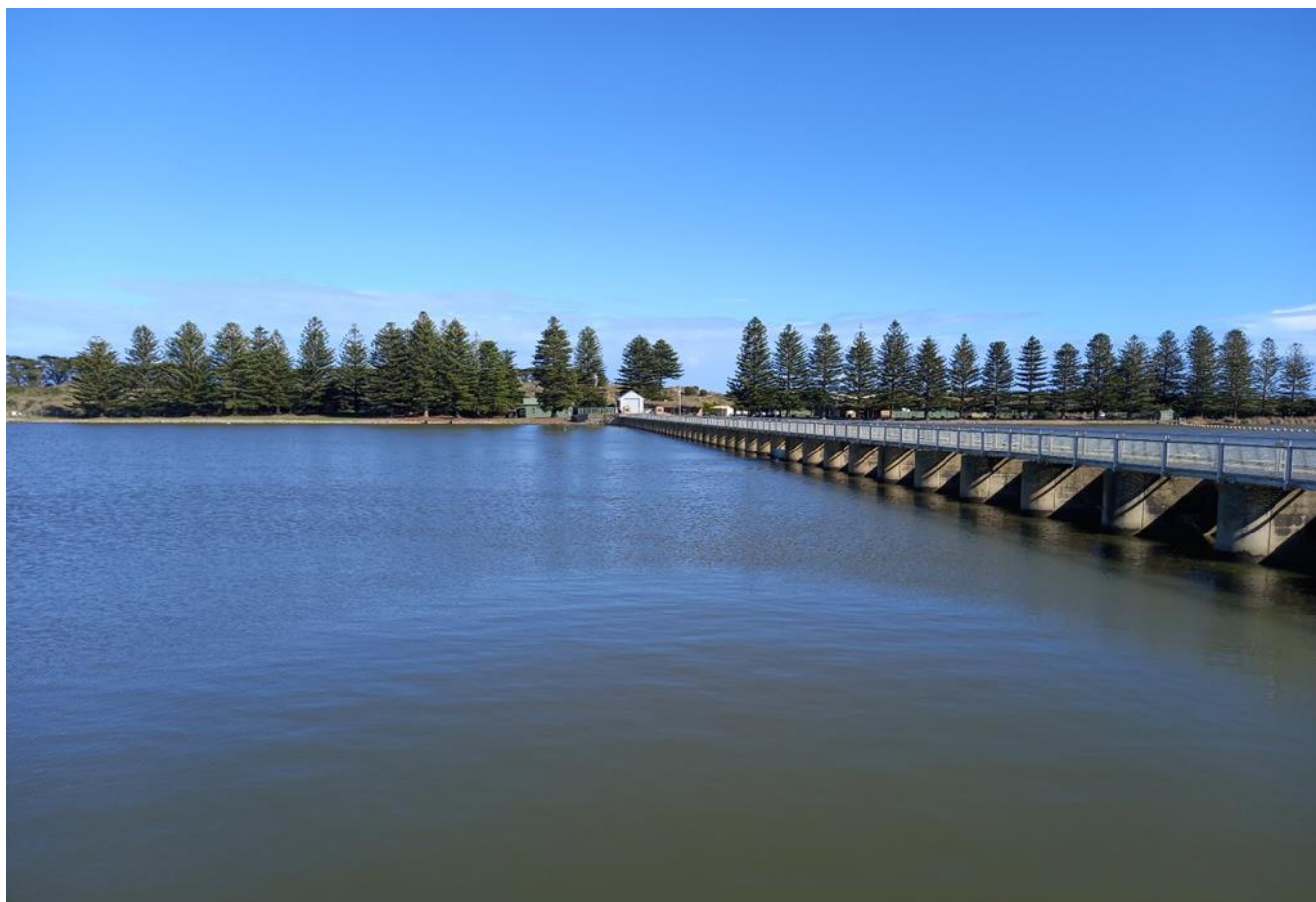
Photo 2 – Goolwa Barrage, one of the South Australian barrages between the Lower Lakes and Coorong, Murray Mouth (Photo courtesy: Jamie Walker, MDBA).
