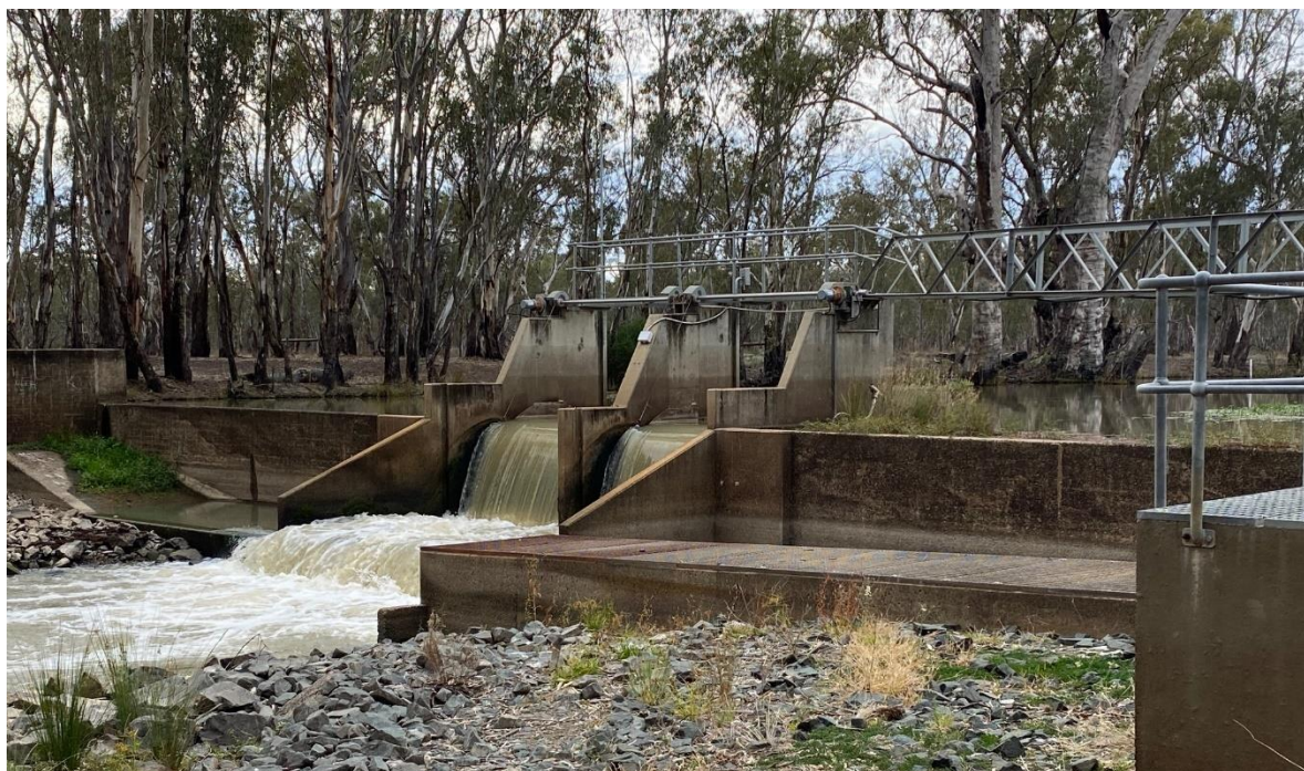
Photo 2: Rices Weir on Broken Creek (Photo courtesy of Jacki Thompson (MDBA))
