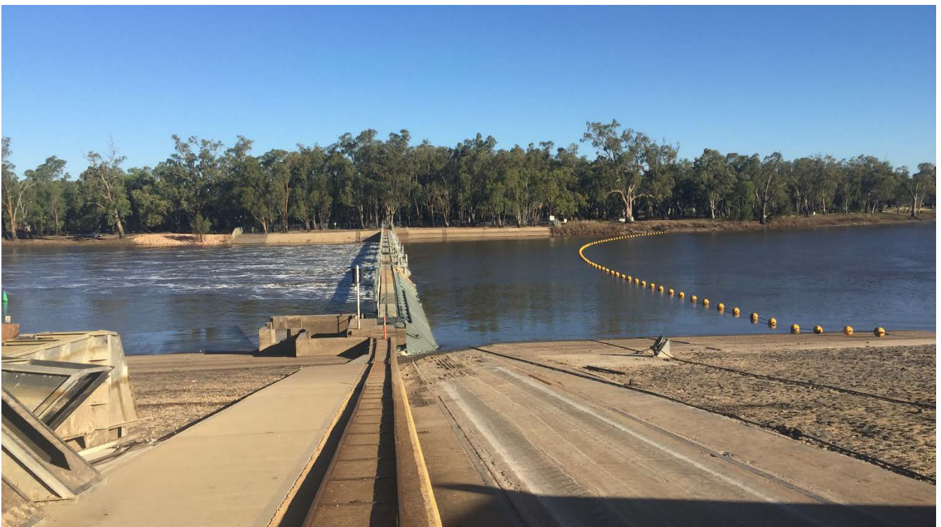
Photo 2 – The Mildura Weir was reinstated over the weekend, and the upstream pool will be raised to near FSL in the next few days. Source: Julian Kelleher, Goulburn-Murray Water.
