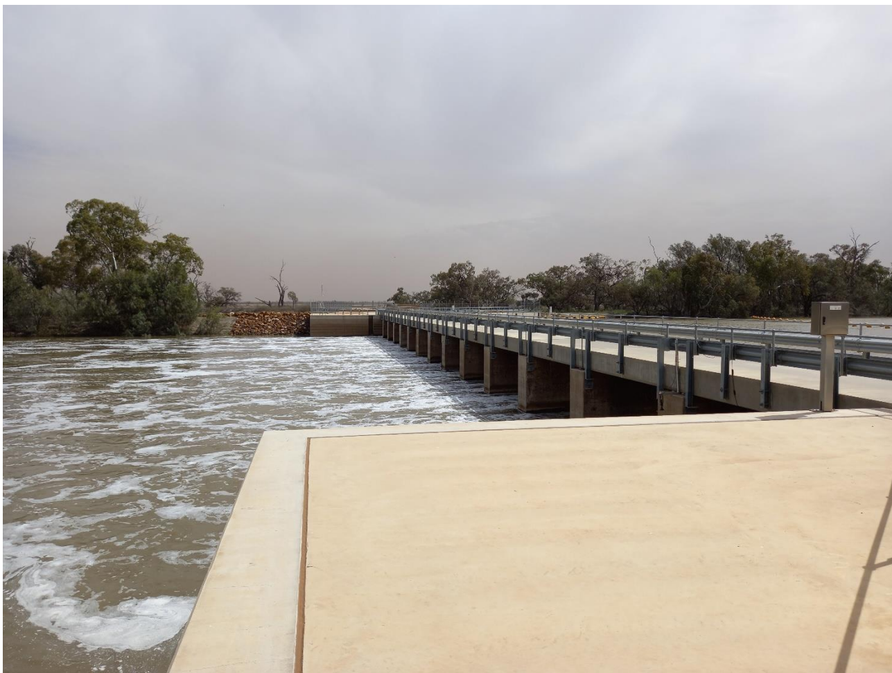
Photo 2: Flows being released from Chowilla environmental regulator to inundate the Chowilla floodplain, photo courtesy Jamie Walker MDBA.
