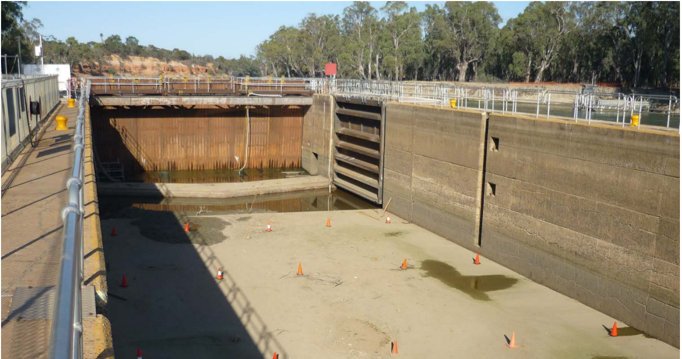
Figure 2 – Lock 15 dewatered to enable refurbishment (Photo: Phil Cocks, Water NSW)
