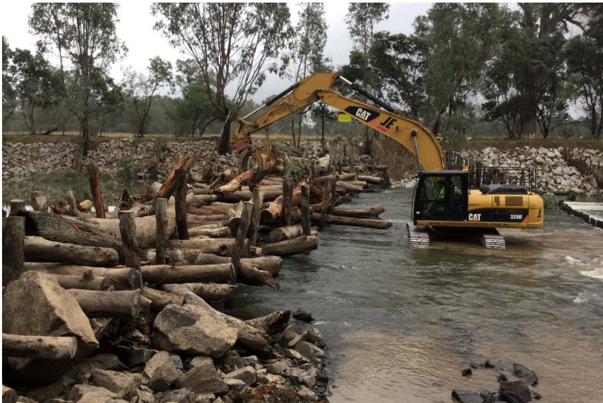
Photo 1 – Log jam construction on Dights Creek, an anabranch of the River Murray, downstream of Hume Reservoir. Source: Ben Berry, NSW Department of Primary Industries
