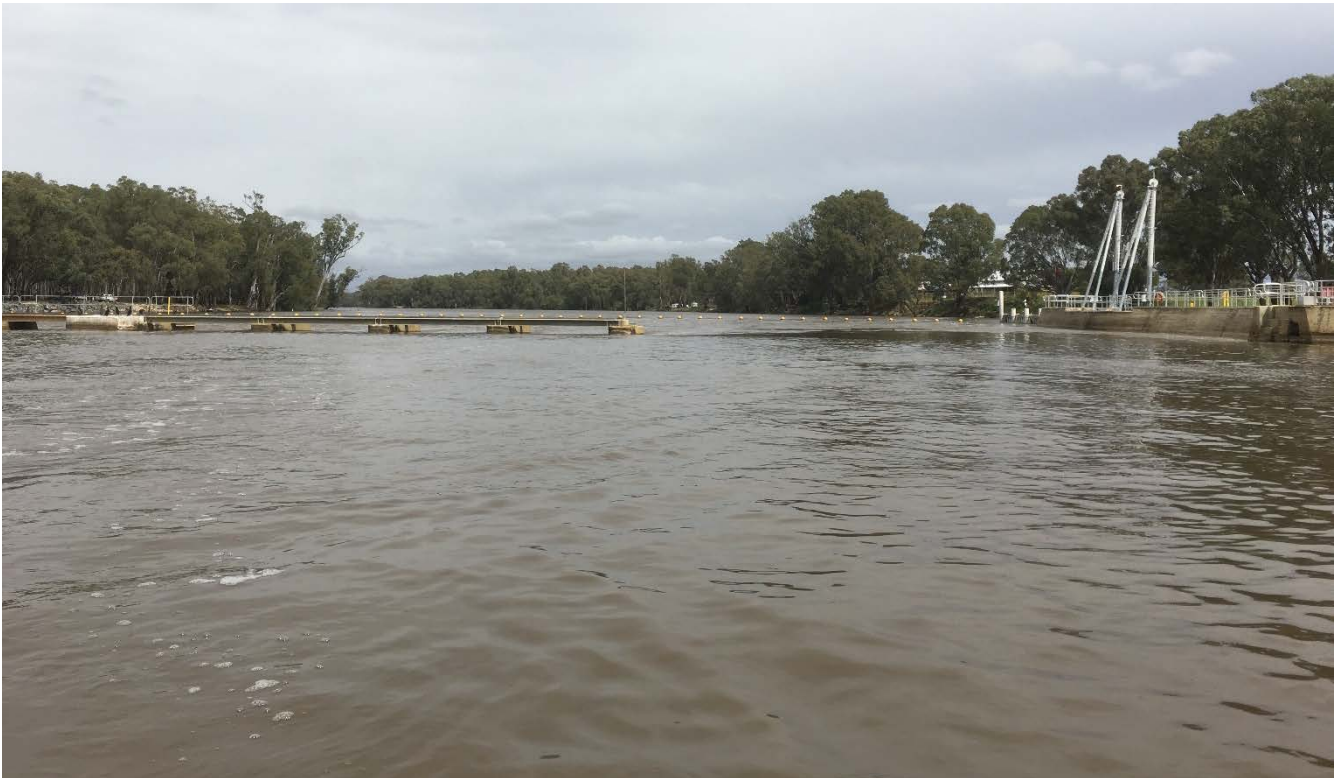
Photo 3 – High flows have resulted in the Wentworth Weir being temporarily removed. Photo: Danny Bourke, WaterNSW.
