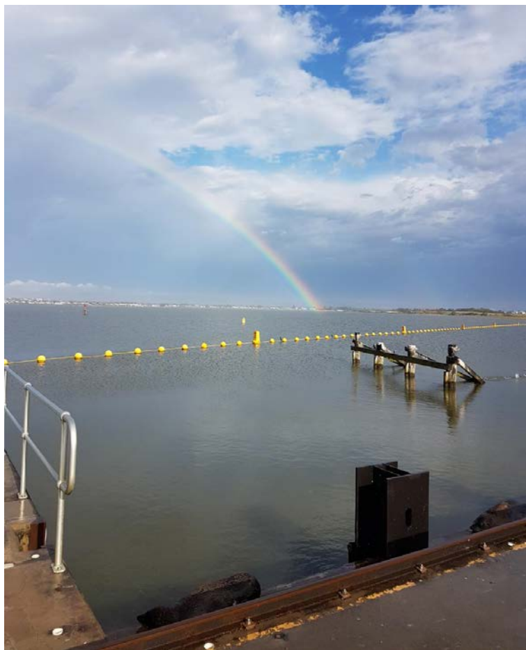
Photo 2: Goolwa Lock looking towards Goolwa (South Australia). Photo: SA Water.
