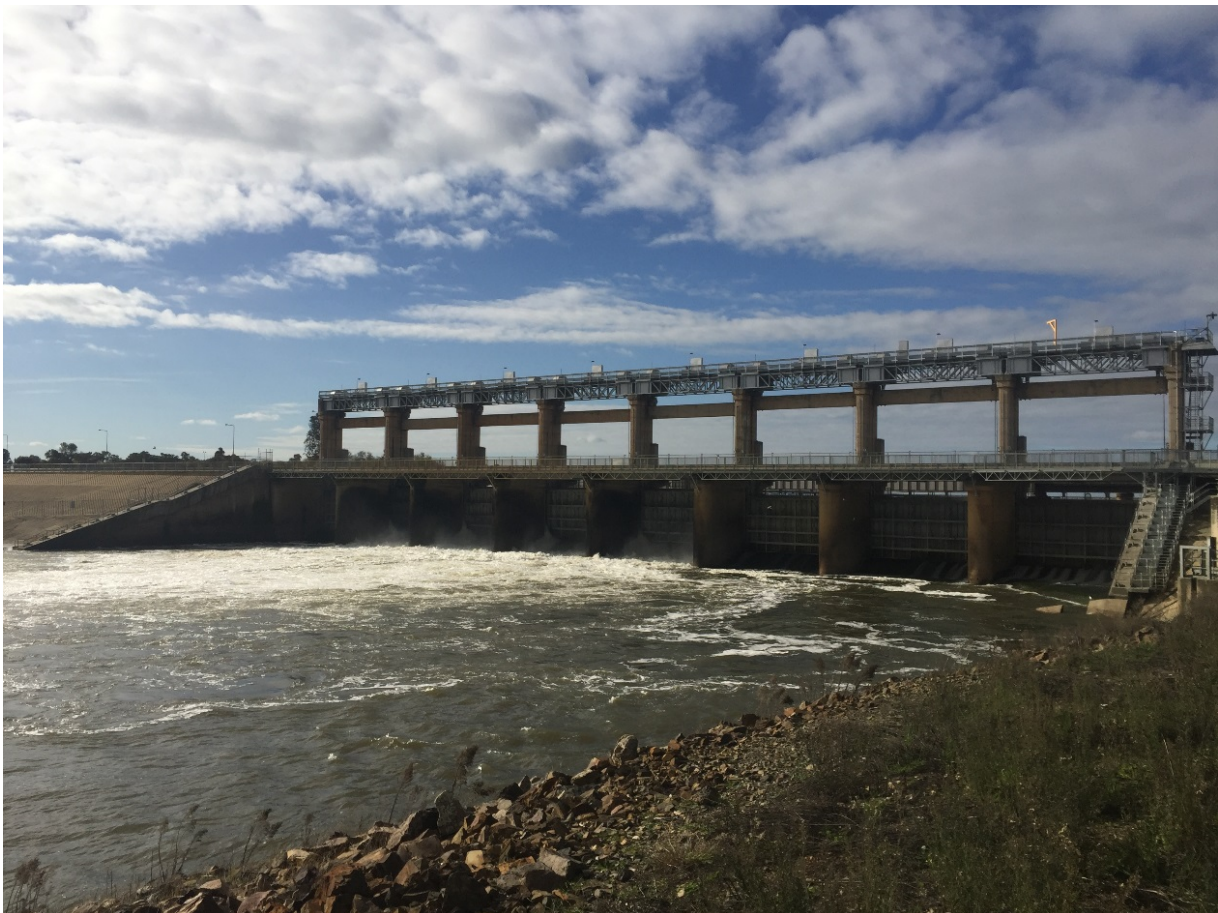
Photo 2 – The release through the gates of Yarrawonga Weir when the flow was 17,400 ML/day on 27 June (Photo courtesy: Brad Moutat, Goulburn-Murray Water)
