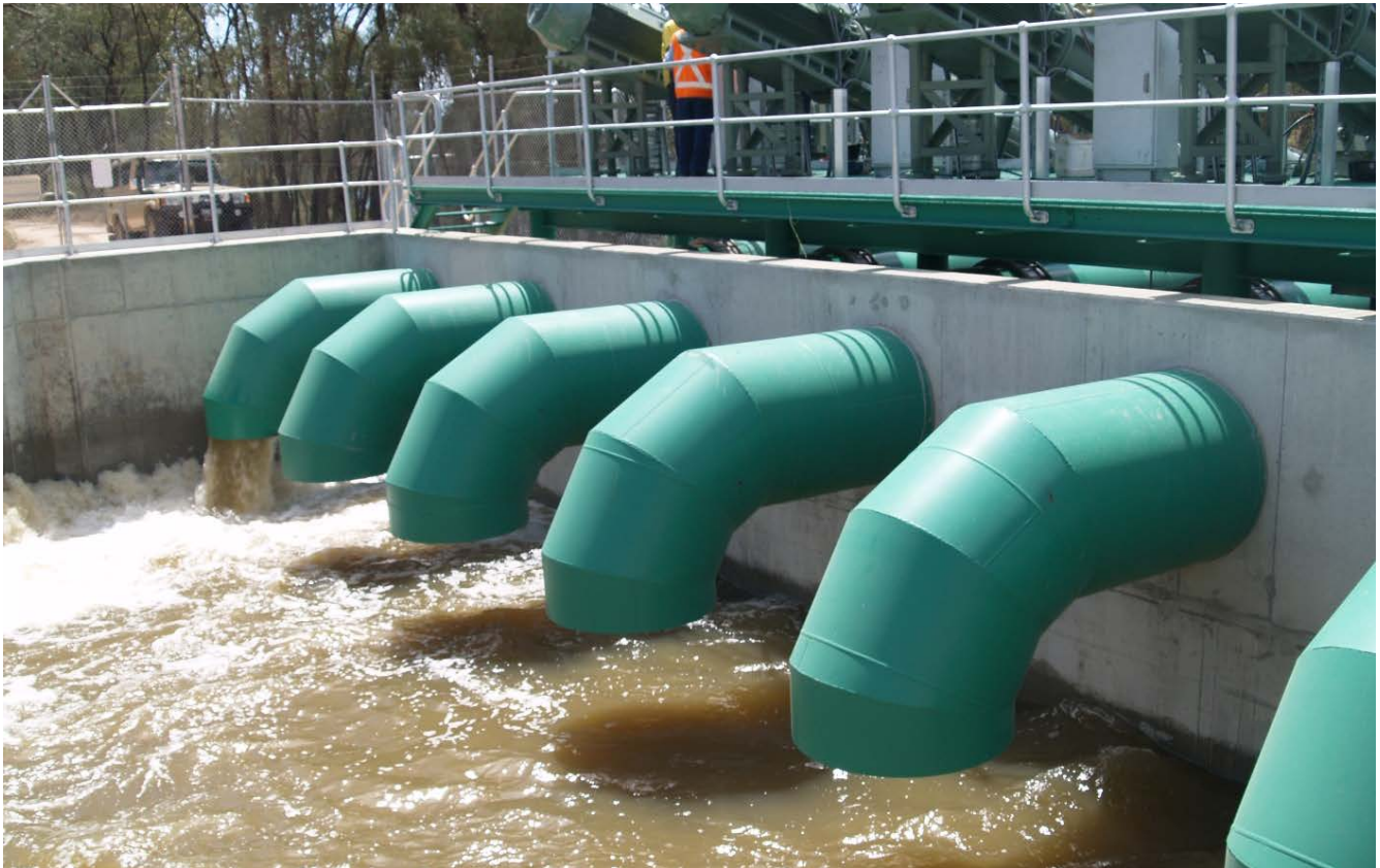
Figure 3 - water passing through the outflow pipes from the pumps that can now supply environmental water to Hattah Lakes. Photo: Heather Peachey, MDBA.
