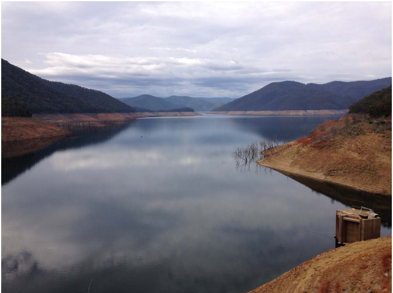
Photo 1 - Dartmouth storage at 43% capacity exposing the top of the high level inlet tower – bottom right of photo (28 April 2016). Photo: Adam McLean, MDBA.
