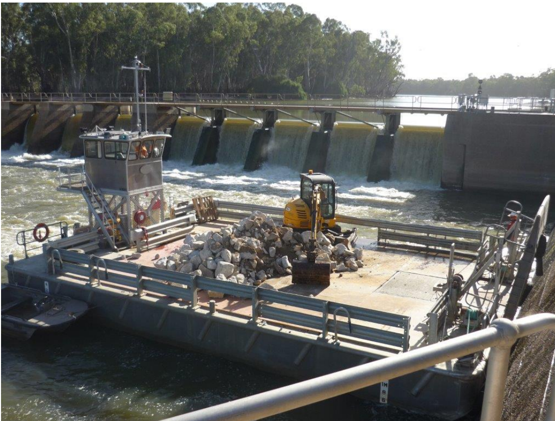
Photo 1– Looking upstream at Euston Weir. The weir pool is currently being varied to manage downstream flows whilst erosion control measures are being undertaken. (Source: Phil Cocks, Water NSW)
