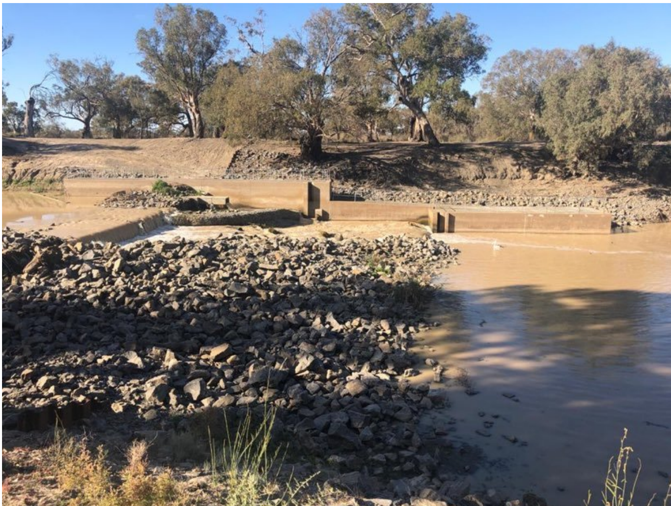
Photo 1: Darling River at Weir 32 (Image courtesy Anita Wilkinson)
