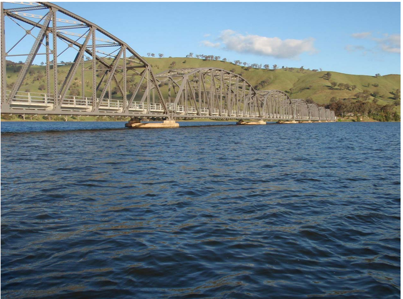
Figure 1 - Bethanga Bridge over Hume Reservoir
