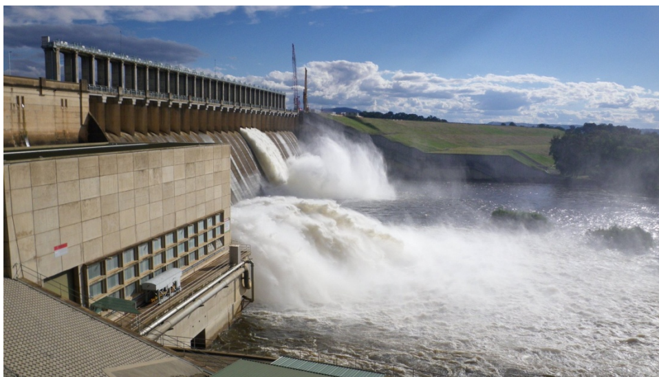
Figure 1 Hume Dam spilling floodwater at a release of 40,000 ML/day, 9th December 2010.
