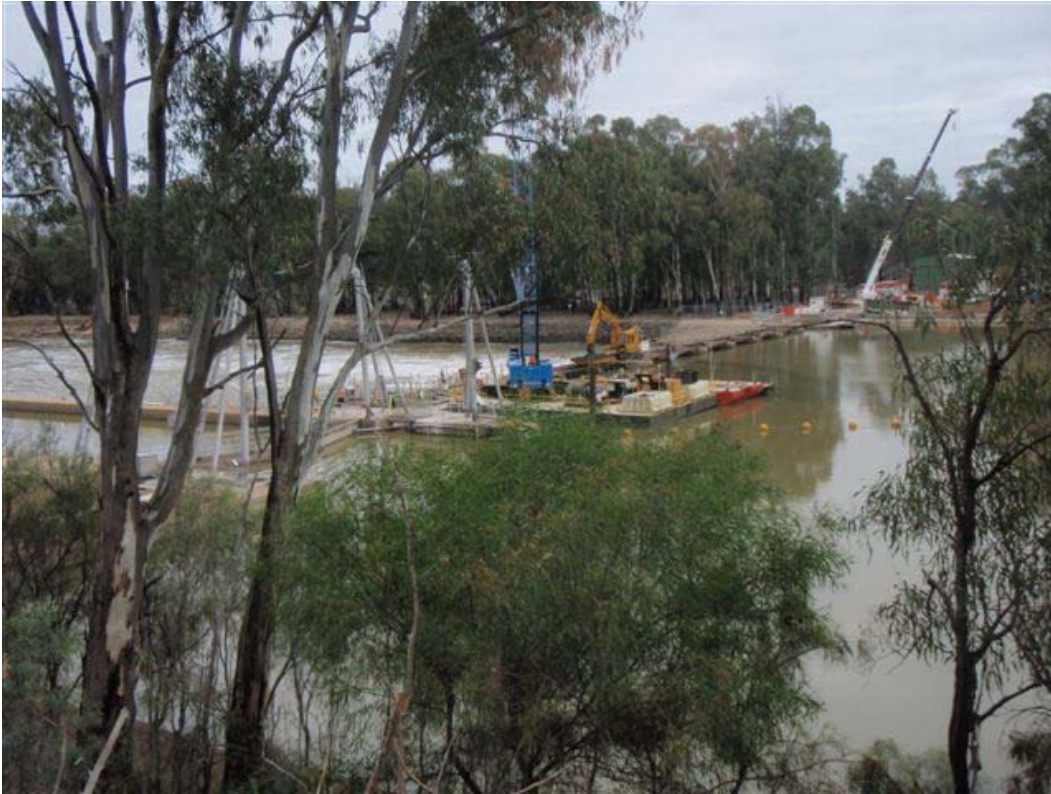
Figure 1 – Construction works at Euston Weir are continuing.
