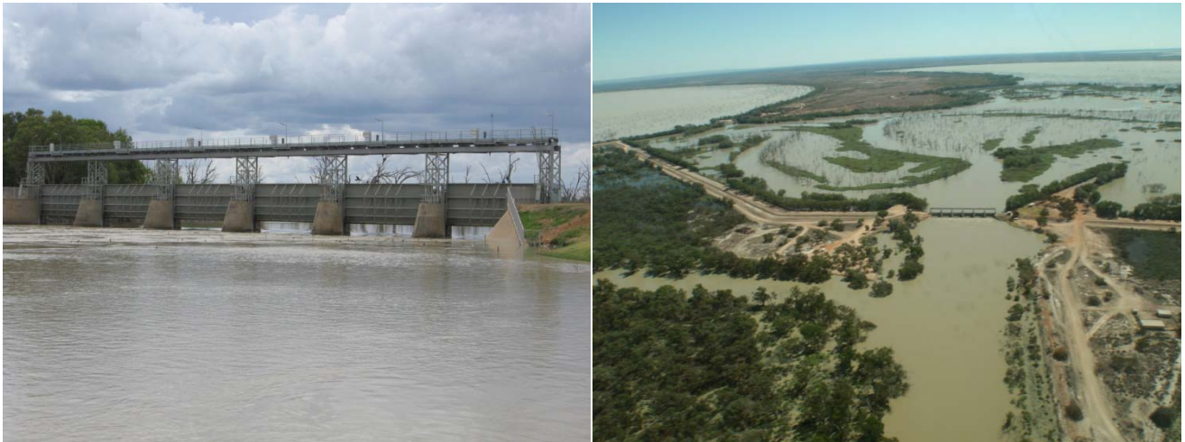
Figure 1 Gates out at Main Weir (Left) and aerial view looking upstream to Main Weir and Lake Wetherell (Right) (Photos provided by Barry Philps (NSW State Water)).
